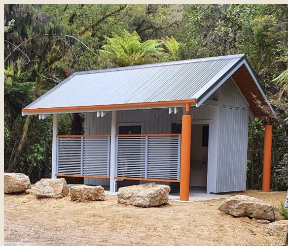
Figure 2- New toilet block Box Canyon car park
